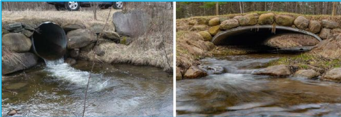
Culvert improvements Ausable River Watershed, NY
