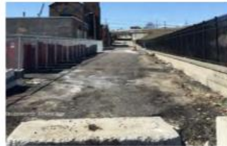
(B) Narrower unpaved portion of the right-of-way extending to the waterfront. This is a narrow stretch with limited vehicle activity.
